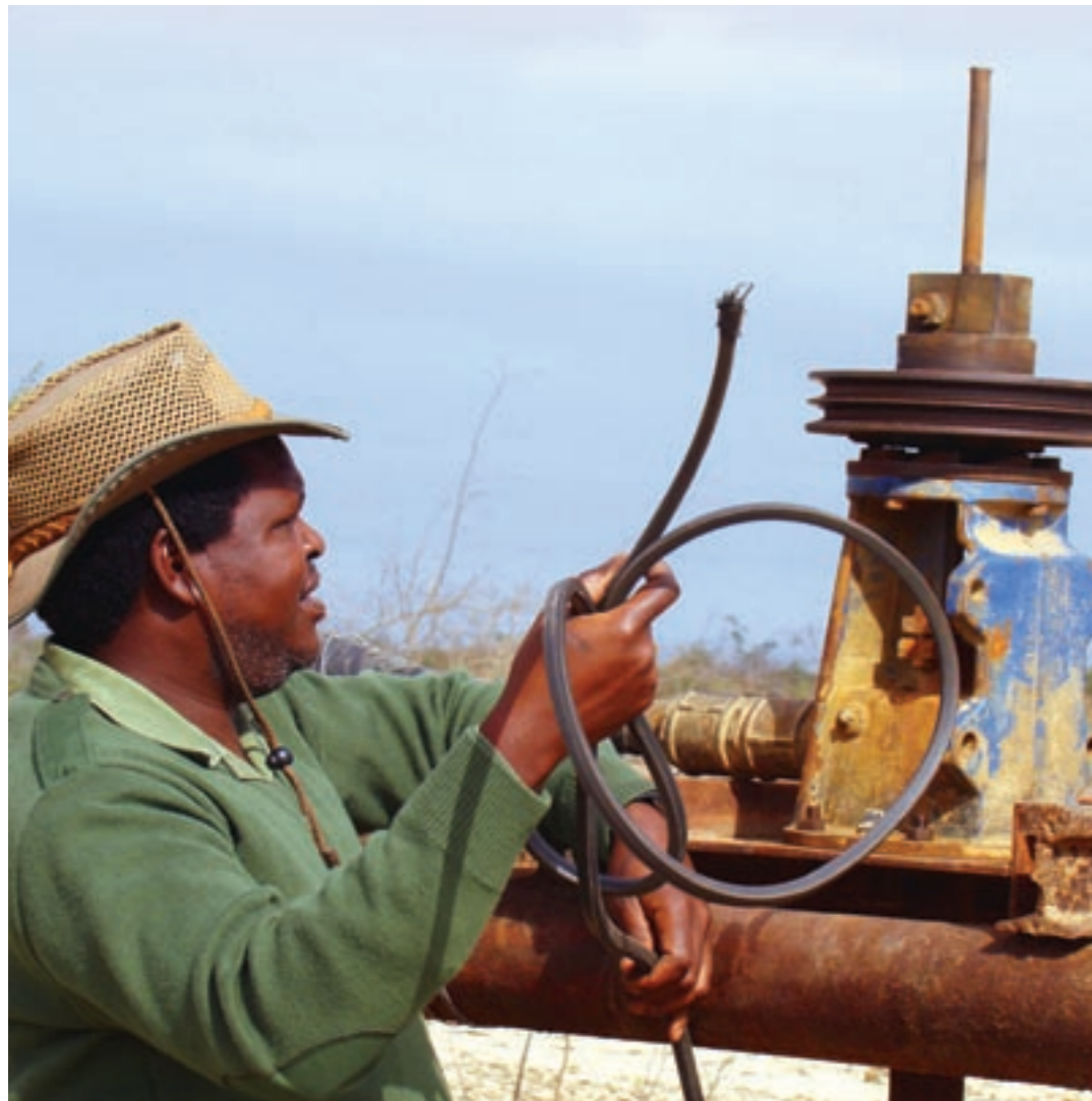
Repairs to water installations is a major activity that requires a dedicated water-maintenance team.
